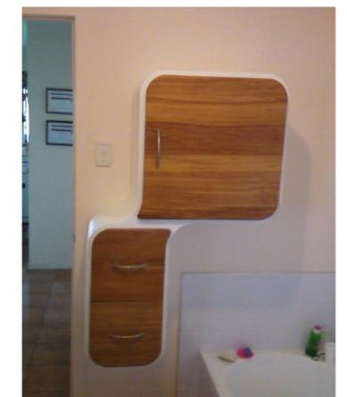
The final job that needed to be done was to screw in the unit to the wall. This job required 3 people, 2 to hold it in place and another to screw the coach bolts into the wall. Now the storage unit is ready to be used by my client.
